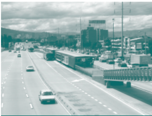
Total segregation of bus lanes from the rest of the traffic, such as what was done for TransMilenio in Bogotá, markedly reduces both emissions and travel time.
