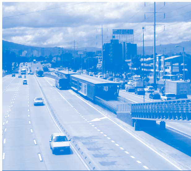
Total segregation of bus lanes from the rest of the traffic, such as what was done for TransMilenio in Bogotá, markedly reduces both emissions and travel time.
