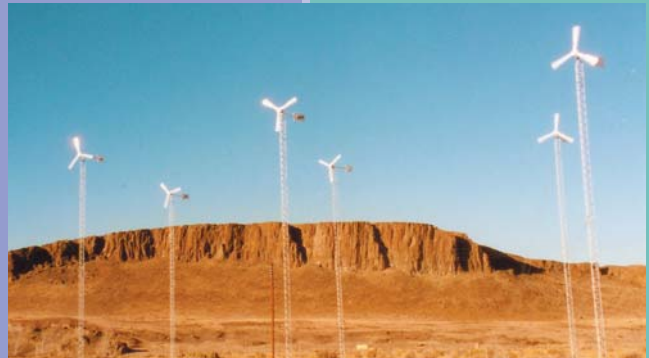
Wind power mini-grid serving a village in Argentina.
