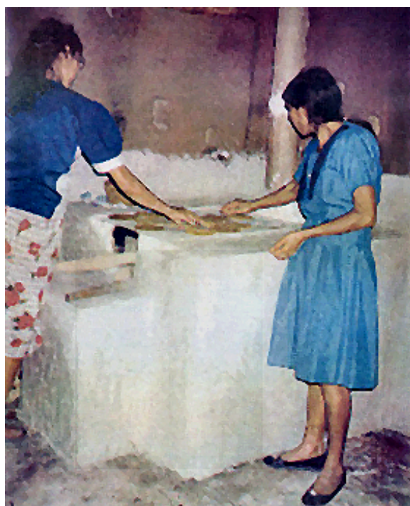
Figure 4.2: The Tezulutla'n improved stove.
