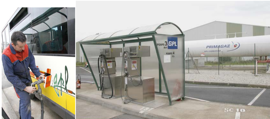
Figure 5: LPG fuelling Station
