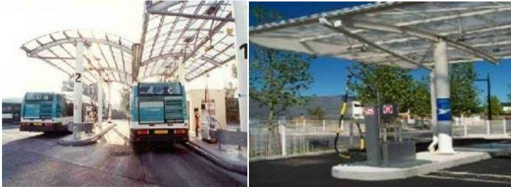
Figure 6: CNG station similar to a fuel diesel station (Creteil depot – France)
