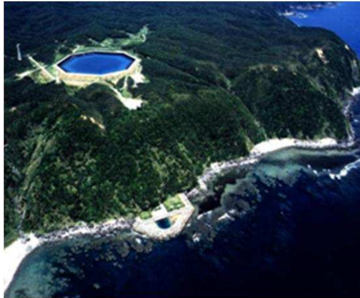
Figure 5-2 Bird's-eye view of a seawater PSP in Okinawa (Japan)
