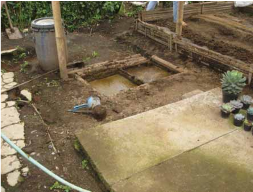
Slurry Overflow Pit: Slurry from the Overflow Pit is Mixed with Soil to make Organic Fertilizer
