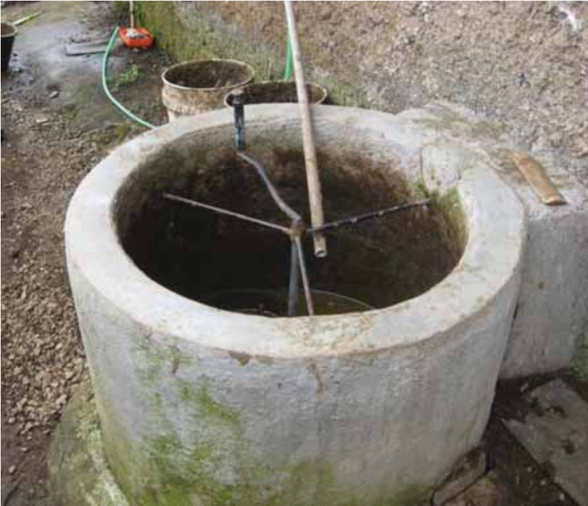
Slurry Mixer Reservoir
