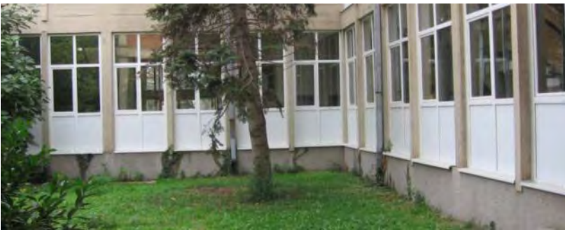
New Thermopane Windows in Skopje School
