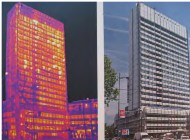
Heat Profile of Administrative Building in Belgrade
