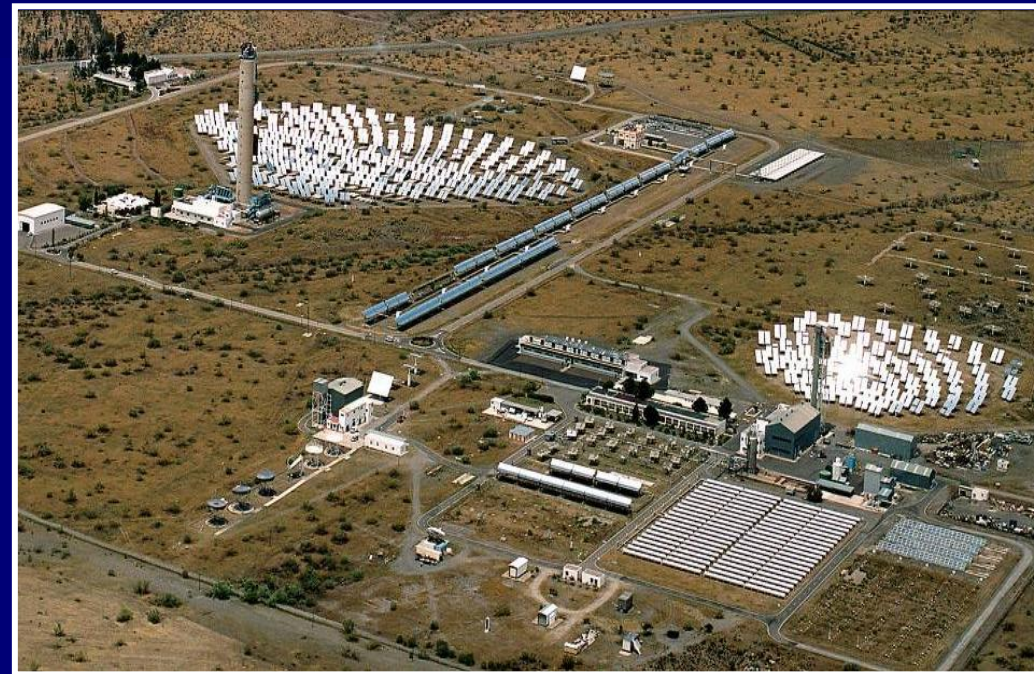
Almeria Solar Platform (PSA) 1978-2011
