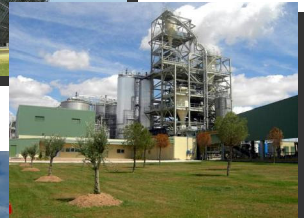
Cellulosic ethanol pilot plant using enzymatic hydrolysis
