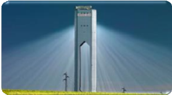
20 MW CSP tower (Spain)
