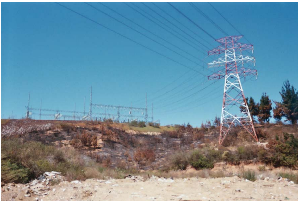
Burned land site near electricity towers. Ruta 68, Valparaíso, Chile.
