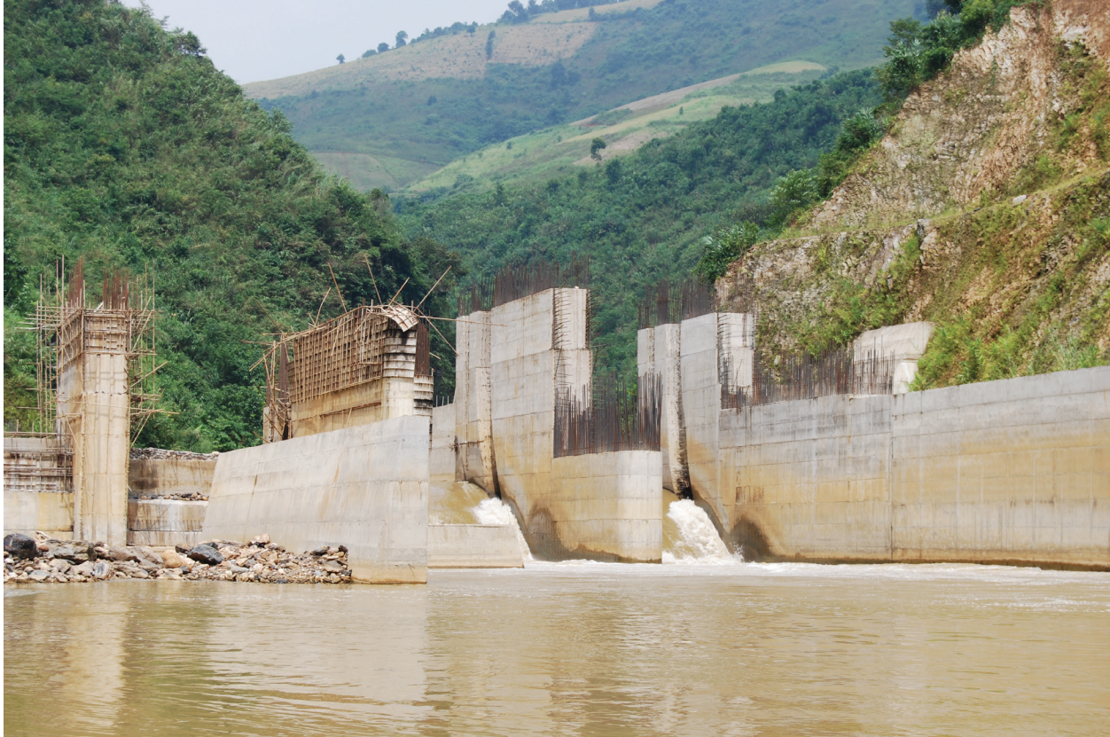
PHOTO 5.1 NAM HOA DAM UNDER CONSTRUCTION
