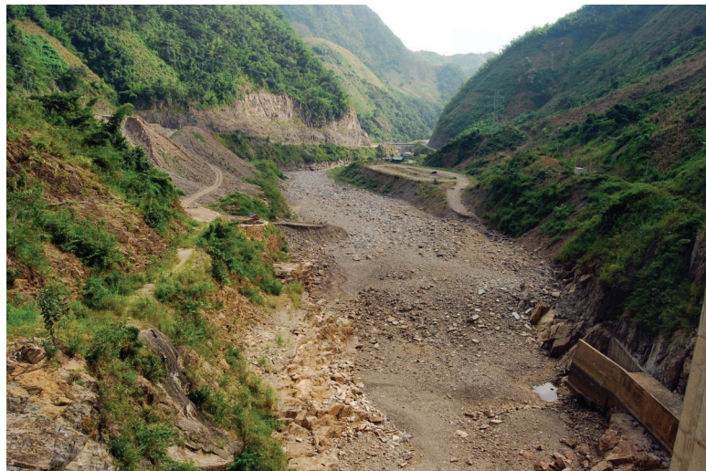
PHOTO 6.2 DRY RIVERBED BELOW NAM CHIEN 2 DAM
