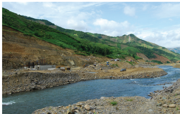
PHOTO 4.1 CONSTRUCTION OF PA CHIEN TUNNEL
