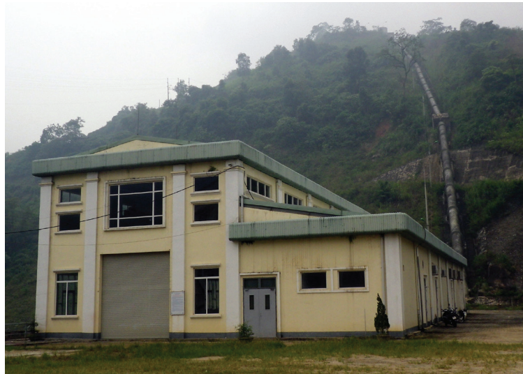
PHOTO 2.1 POWERHOUSE AT NGOI XAN 1 SMALL-SCALE HYDROPOWER PLANT
