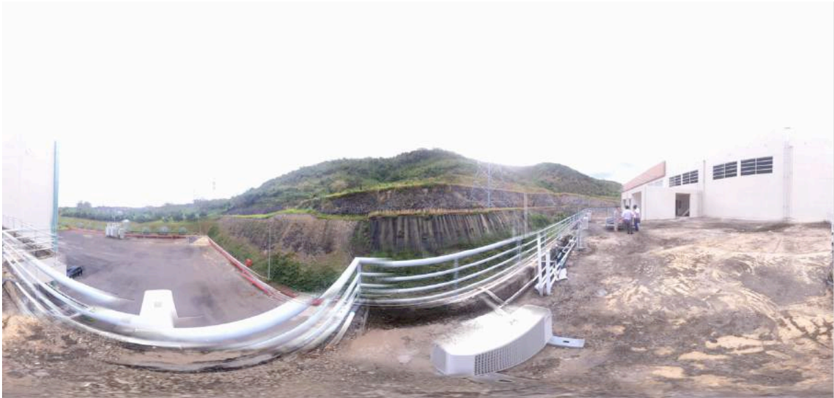
Figure 25: Location on roof of turbine house at river (VNCE2).
