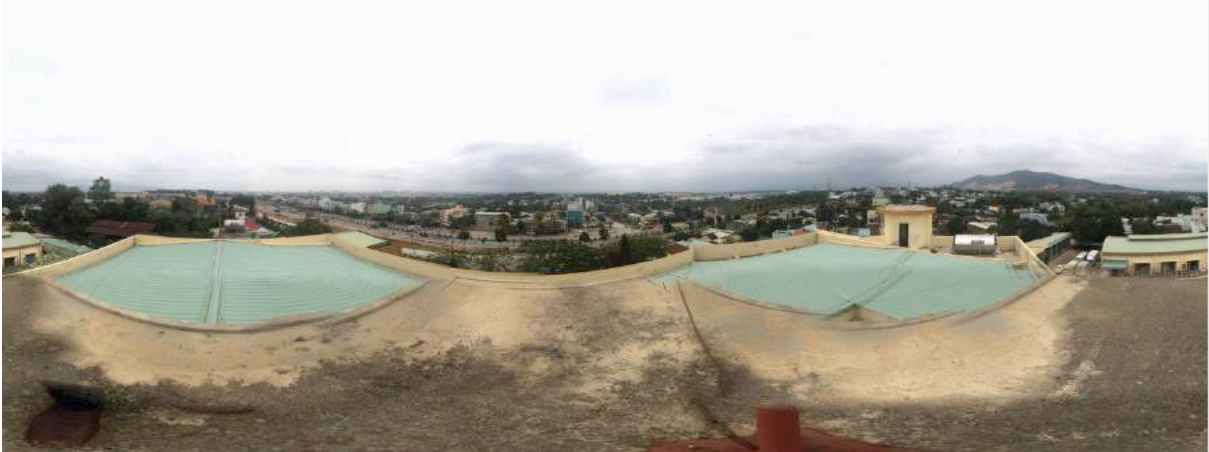
Figure 14: Location at Da Nang region, roof on EVN/CPC rooftop (VNDA1).
