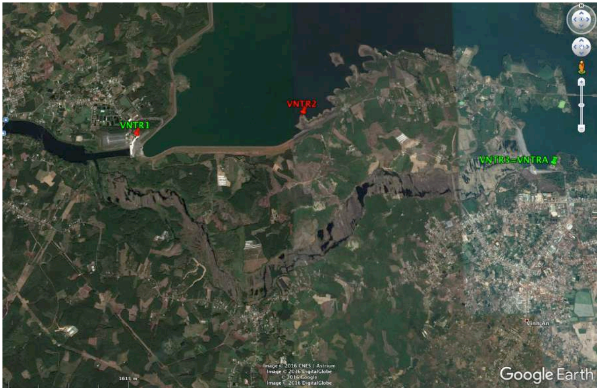
Figure 35: Options for measurement location at Tri An dam
