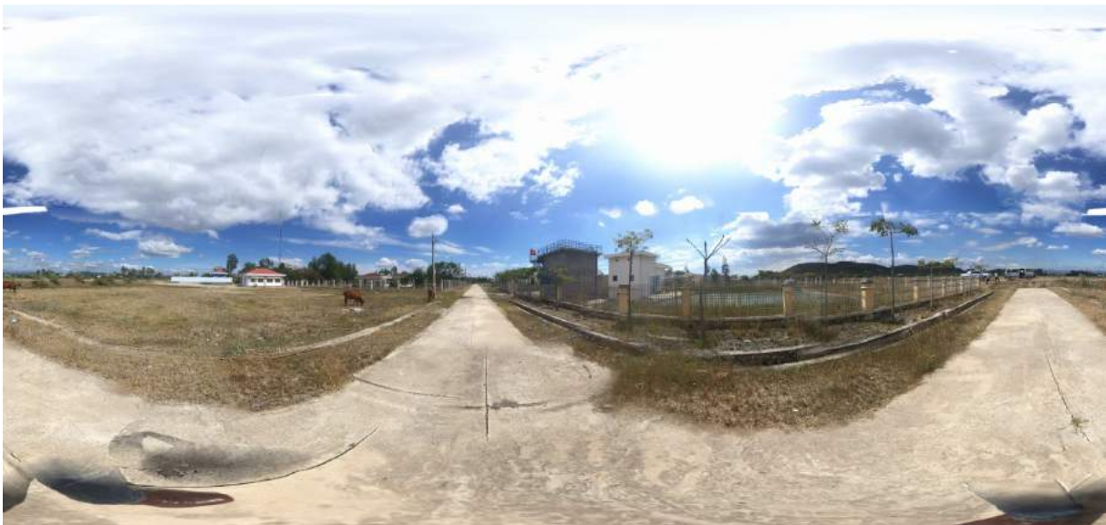
Figure 33: Song Binh, water treatment facility
