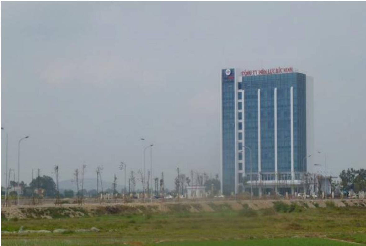
Figure 6: New building of EVN with spacious rooftop and fully flat horizon (VNHA1)
