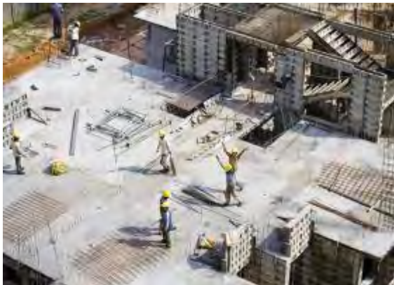
Concrete formwork technology allows rapid construction and also has lower embodied impact than bricks
